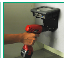
2: Select the position to mount stand kit
